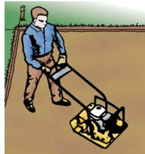
To ensure adequate compaction, you will need to install the base in lifts (layers). If you will be using a hand-tamper, spread an even layer of gravel about 2" thick. If using a plate compactor, you can spread the gravel in 3" to 4" layers.
